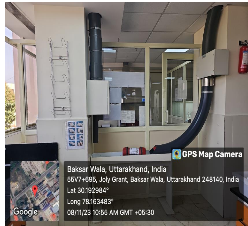
Pneumatic shoot system in the Bacteriology Section
