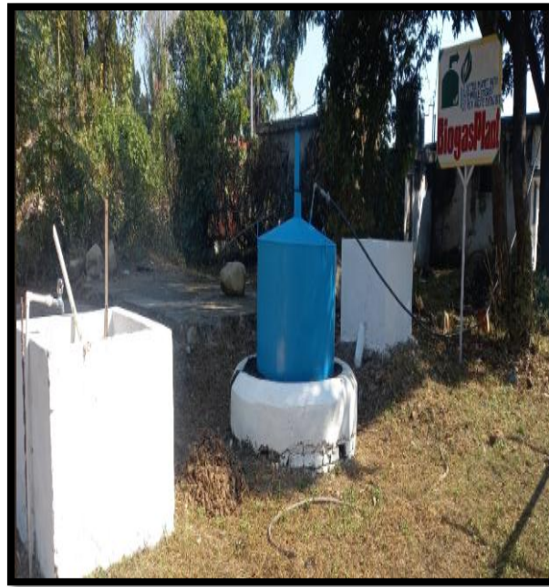
Figure 7.4. Bio-gas Plant of capacity 4 cum/day
