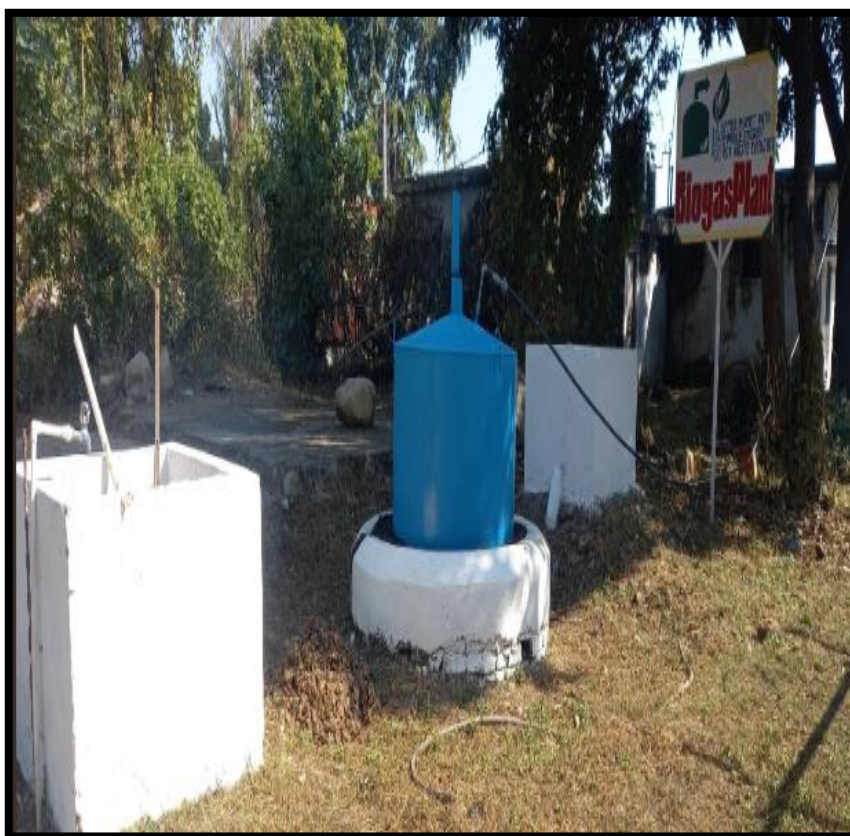
Figure 4.2. Bio-gas Plant of capacity 4 cum/day
