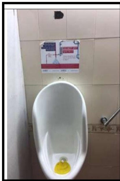
Figure 3.4. Waterless urinals (200 Nos.)
