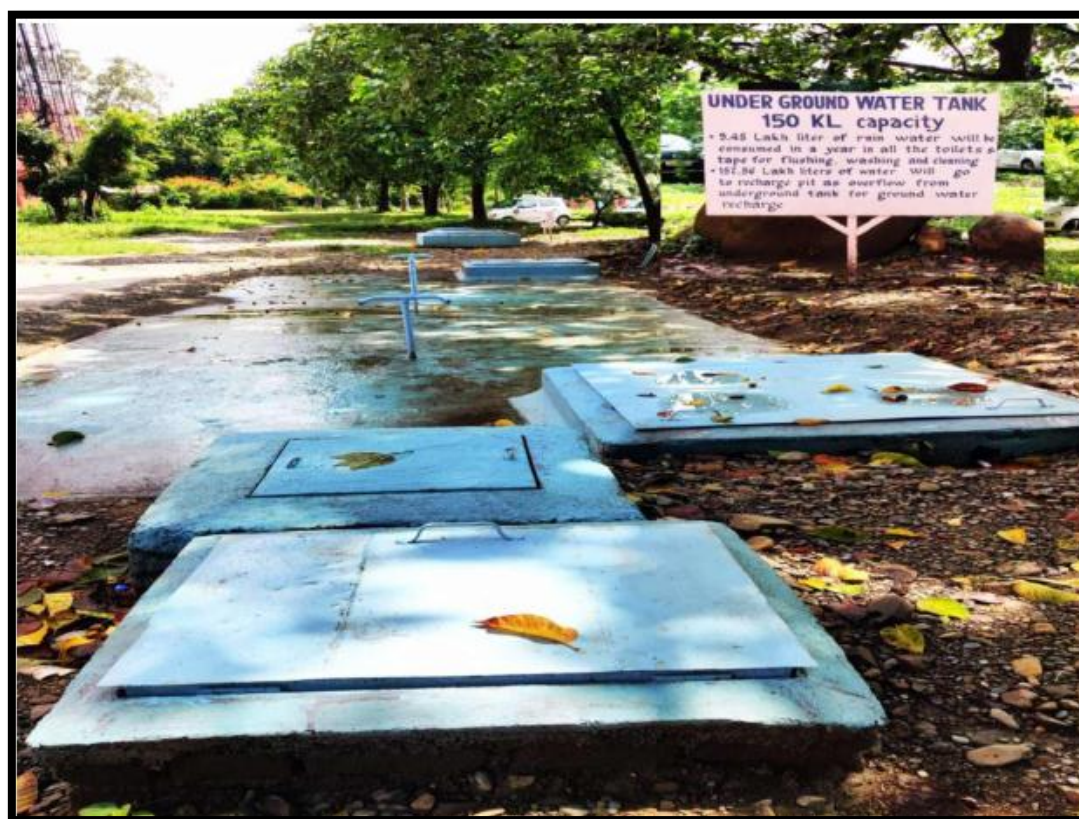
Figure 3.3. Rainwater recharge pit and Underground water tank of 150 KL capacity
