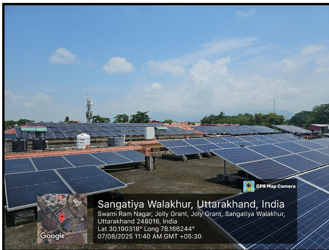
Figure 7.3. Solar Power System installed at SRHU (2.5 MW)
