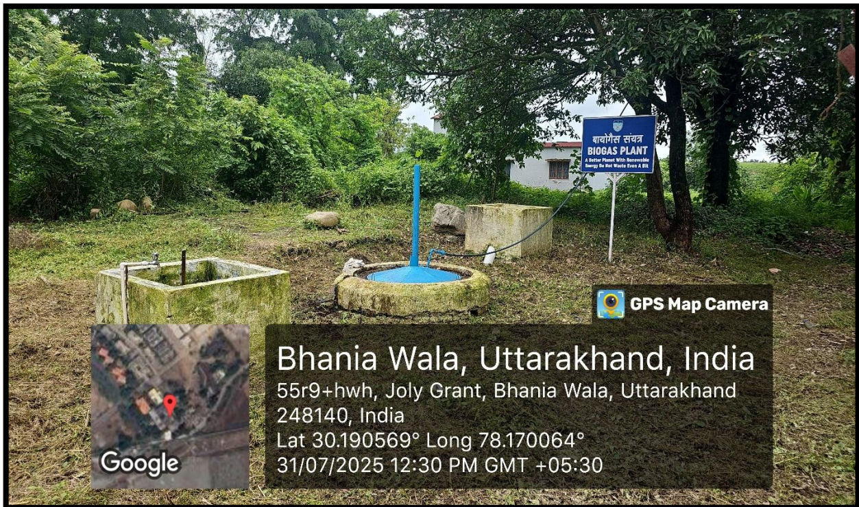
Figure 4.2. Bio-gas Plant of capacity 4 cum/day
