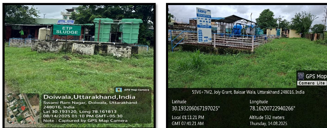
Figure 3.2. ETPs of capacity 90 KLD (40 KLD and 50 KLD) and STP of capacity 1 MLD
