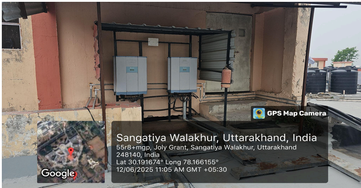
Solar PV plant on- grid inverter for wheeling to the grid
