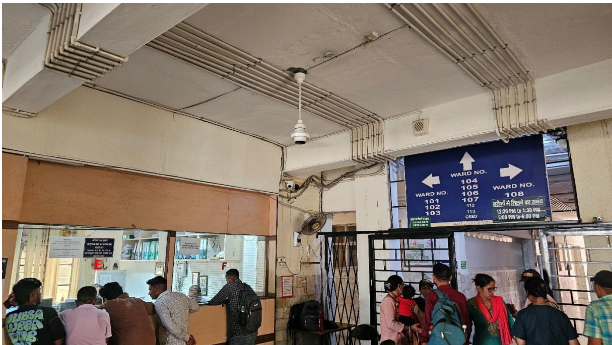
Energy-efficient BLDC (Brushless Direct Current) fans within hospital premises to enhance energy conservation
