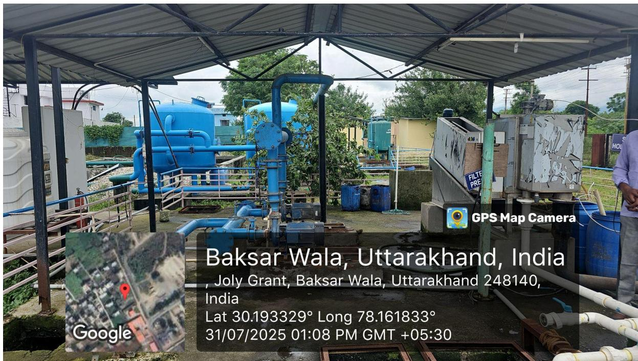
**Filtration tanks, pumps, and sludge filter press at STP, forming part of the advanced wastewater treatment and recycling system**
