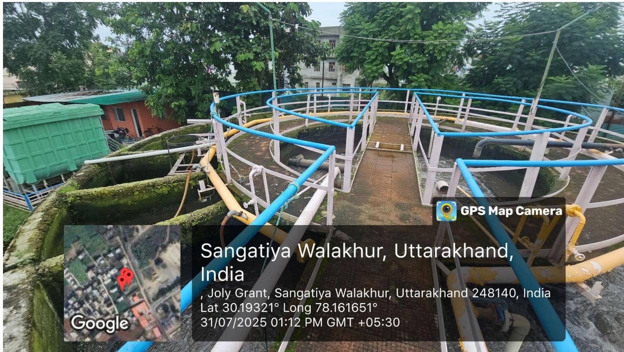
Aeration tank at STP, where wastewater undergoes biological treatment
