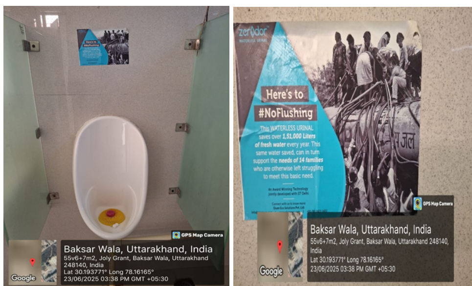
Waterless urinals present at different locations across the University
