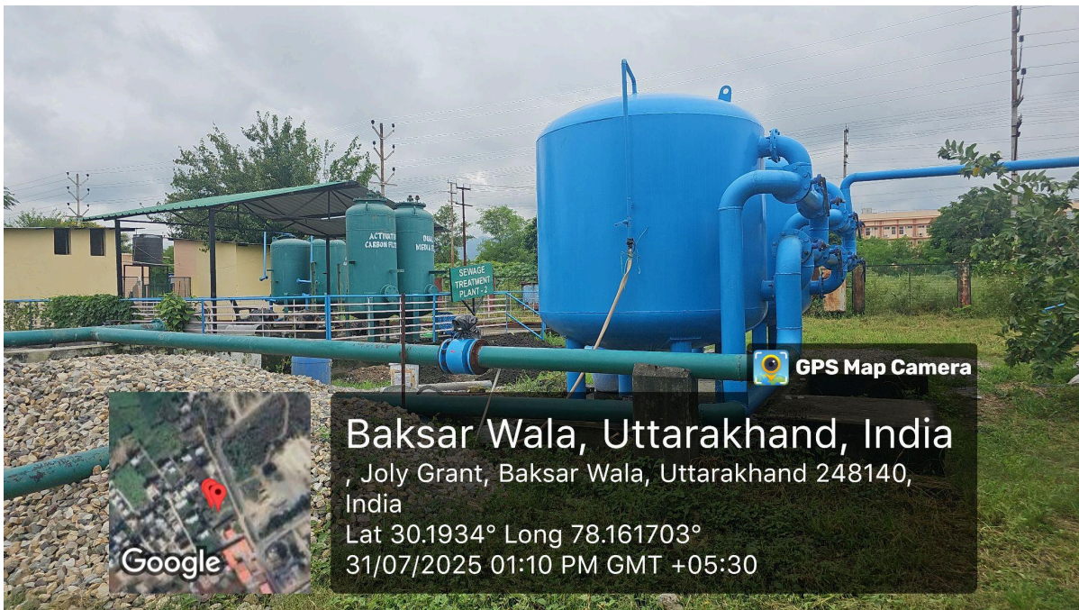
Activated carbon and dual media filters in operation for advanced wastewater treatment
