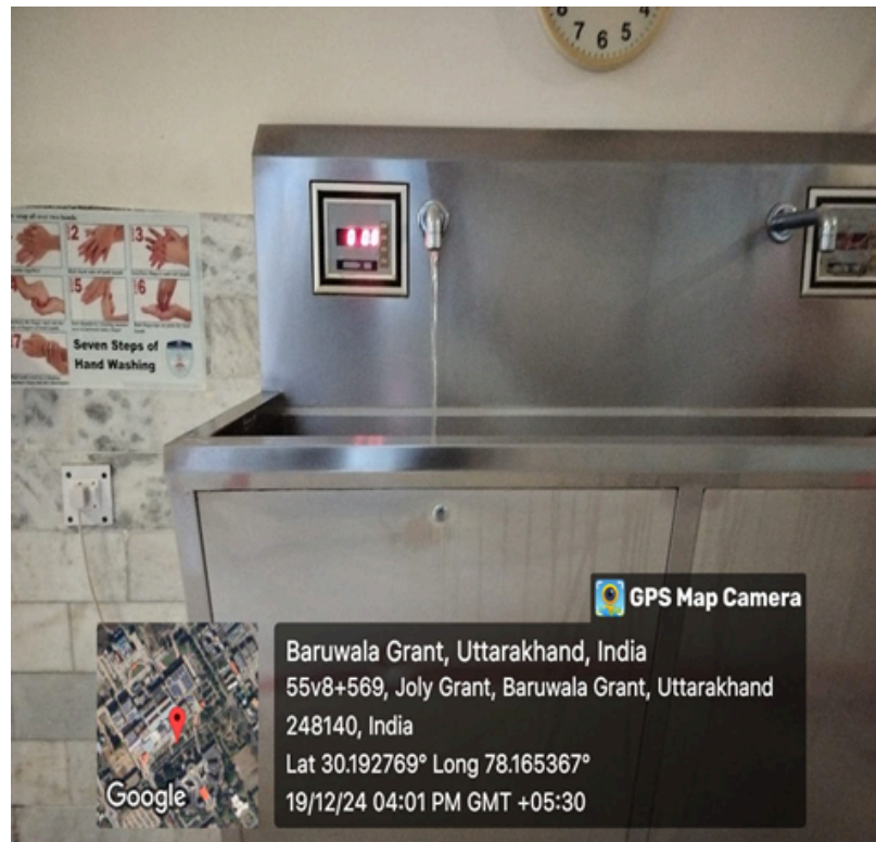
Sensor activated scrub station aiding in water conservation
