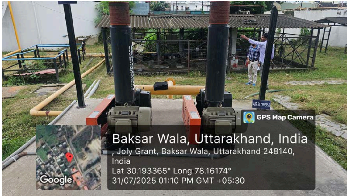
High-capacity air blowers in operation to support the aeration process
