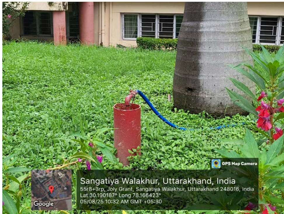
Red-marked tap supplying treated wastewater from the sewage treatment plant, promoting sustainable water reuse for landscaping and greenery maintenance
