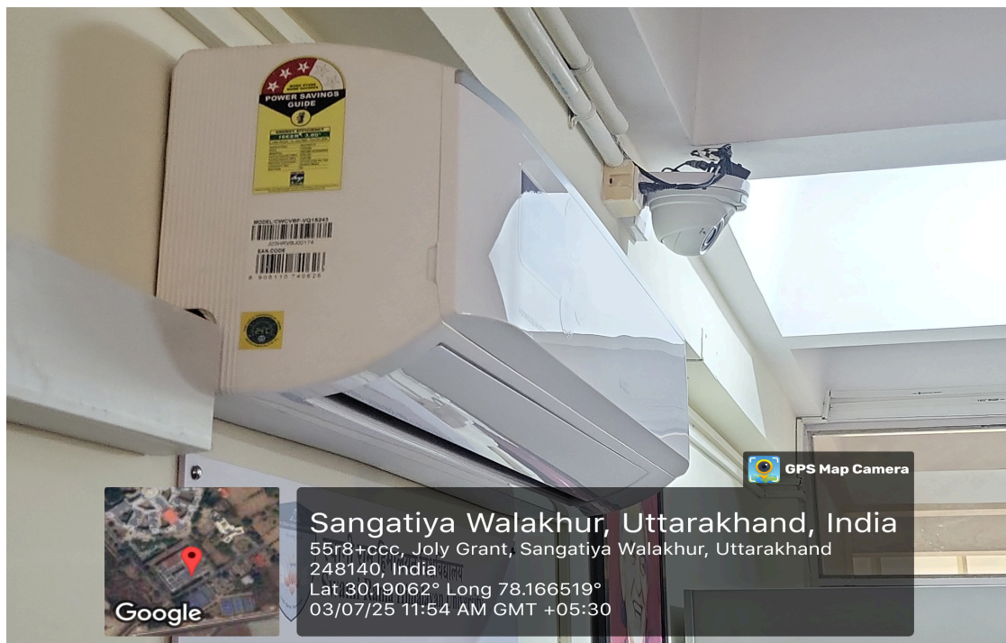
Energy Efficient split inverter air conditioners
