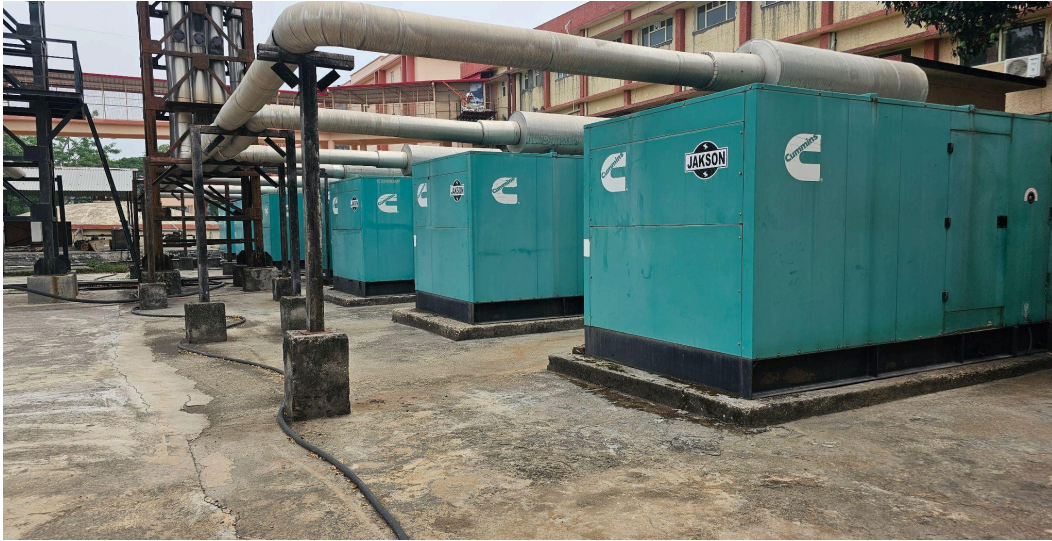
9 Diesel generator sets with Automatic Mains Failure panels and load synchronization system
