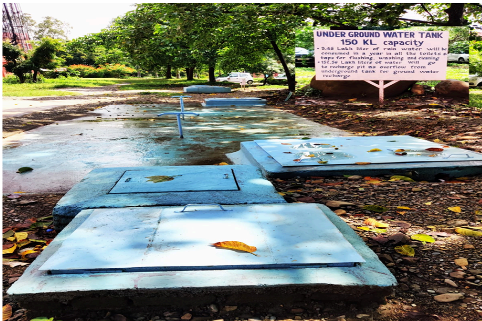
Underground RWH tank (capacity 150 KL)
