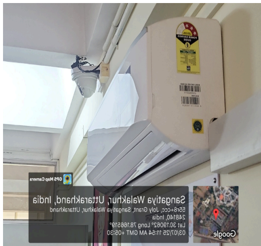
Energy Efficient split inverter air conditioners
