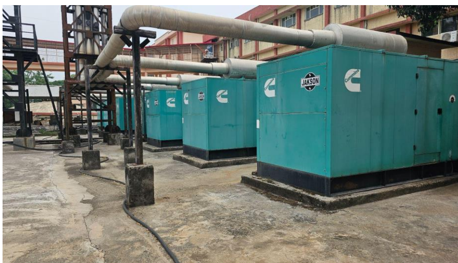
9 Diesel generator sets with Automatic Mains Failure panels and load synchronization system
